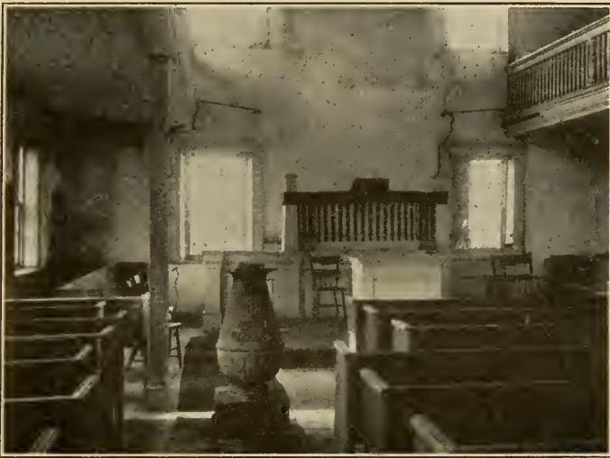
INTERIOR PINE HILL "UNION" CHURCH (About to be torn down)
